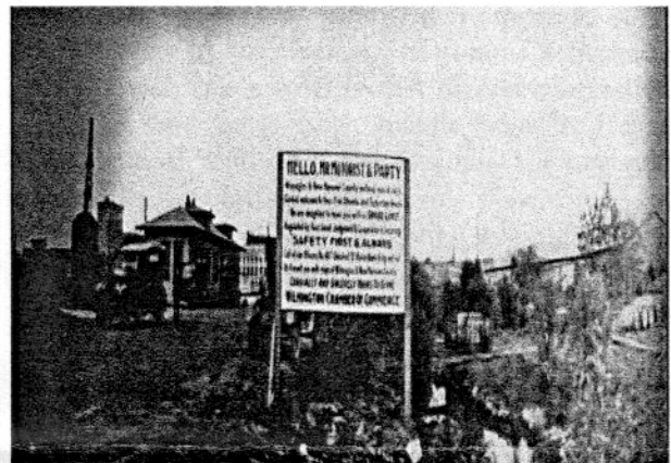
Eagles Island Ferry Landing
