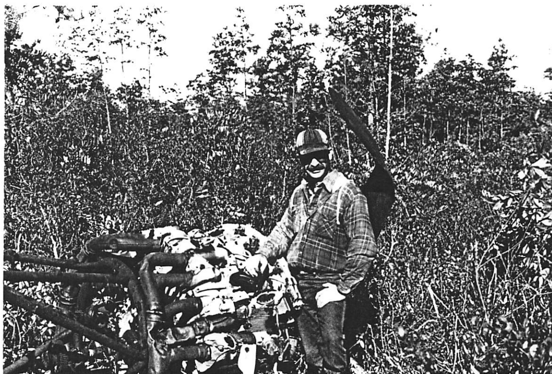
view of motor (Looking North)
