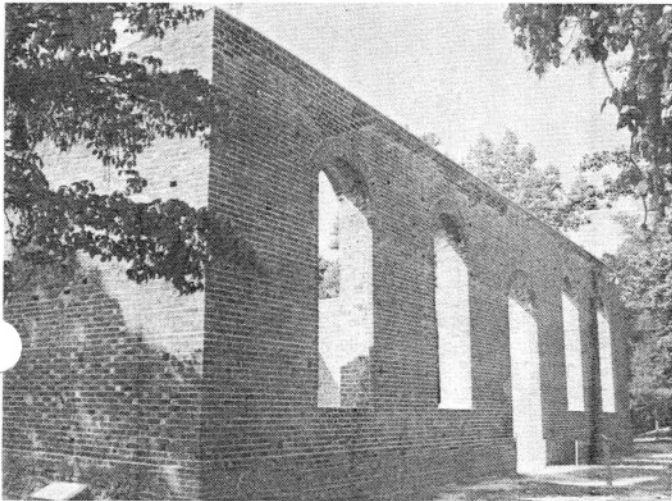
St. Phillip's Church - Stabilized.
