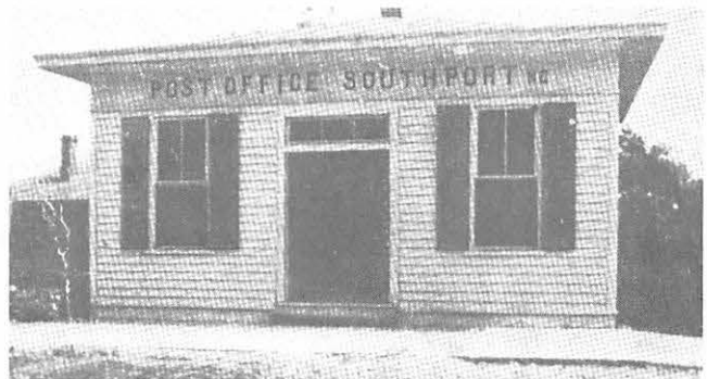
Photo of old Southport postoffice in 1909. This building is still standing and a second floor has been added.
